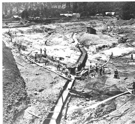
Figure 3. Gravel deposits were washed into sluices (from center to lower part of figure) where gold was recovered.
