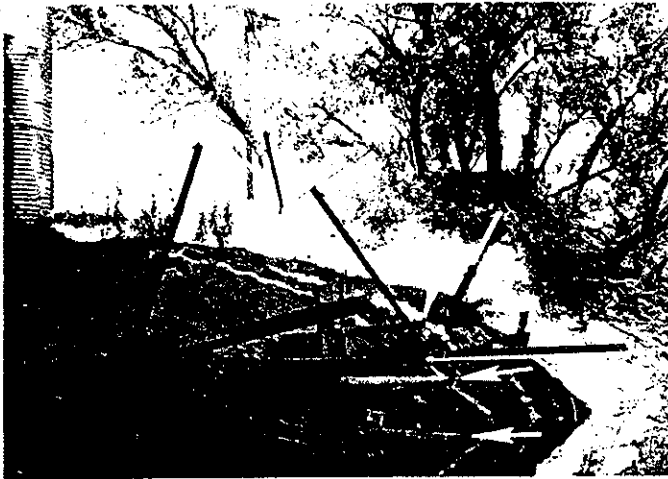
FIGURE 6.—Degradation represented by successively lower water-intake pipes for streamflow-gaging station 2.6 kilometers downstream from Fort Supply Dam, Wolf Creek, Oklahoma. Dam was closed in 1942; photograph was taken in 1951.
