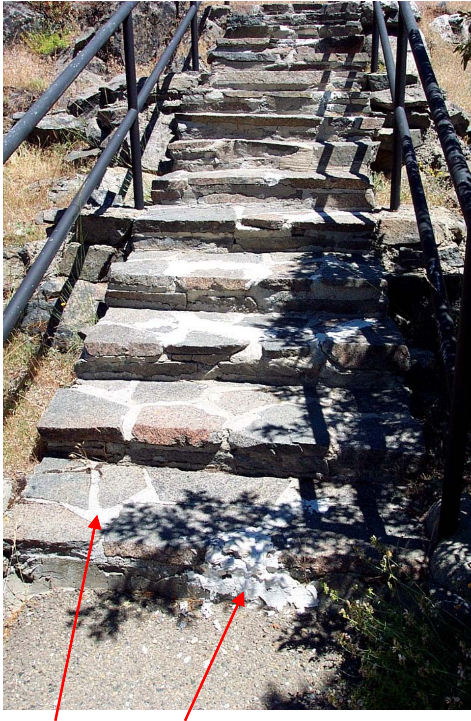
Photo 1. Original grout and repair material on the stairs to the Hell Hole Reservoir Overlook.
