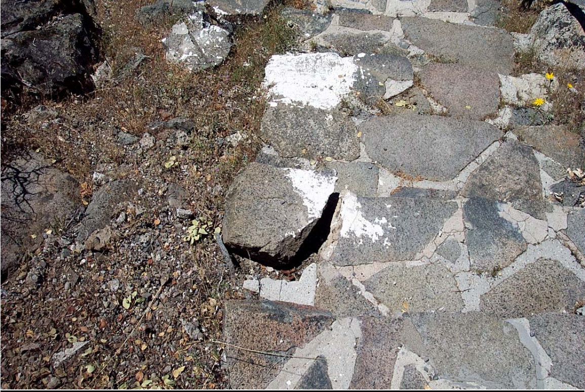
Photo 2. Loose paving stone on the Hell Hole Reservoir Overlook stairs.
