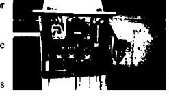
Recommendation: Holes should be filled and gaskets replaced to protect the interior devices from the elements. Conduits should be properly grounded and sealed. The gate position signals should be connected using twisted shielded cables run in a conduit dedicated for instrument signals. Cabinets should be cleaned. Refer to Section 3.2. Drawing 241-08-205 for additional recommendations.
