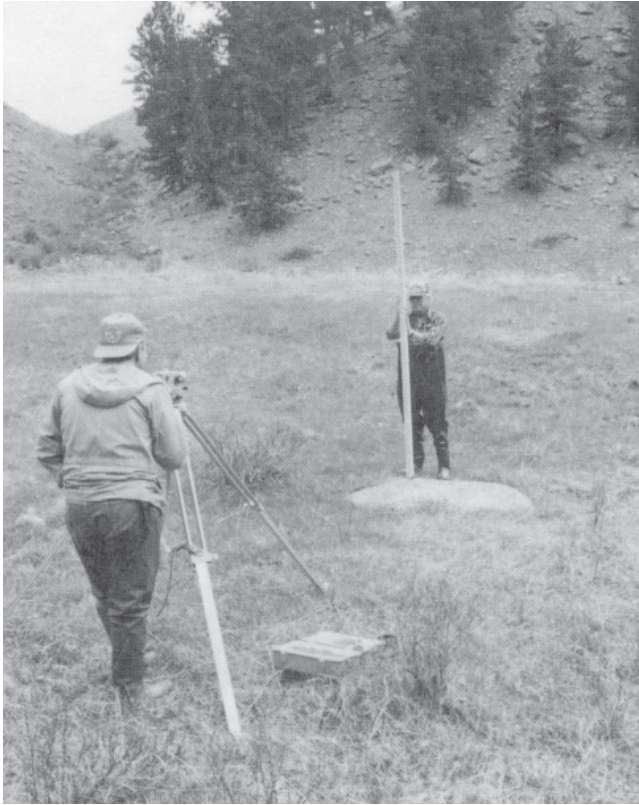
Figure 34. Shooting the elevation of the benchmark.
