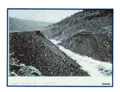
At 9:30 AM on December 23rd, a gully had been eroded across the crest of the dam, and the reservoir began to spill over the top of the fill. When this happened the velocity of flow and the rate of erosion increased rapidly, and soon a major portion of the embankment was washed away and the reservoir was emptied.
