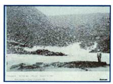
This photo shows the water emerging from the toe of the downstream rockfill shell at 3 PM on December 22, 1964. Some rock has been eroded.
