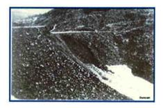
By 7 AM on December 23rd, the flow had increased as the reservoir rose behind the dam, and a considerable portion of the downstream slope had been eroded away.
