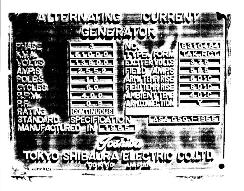
PLACER COUNTY WATER AGENCY MIDDLE FORK AMERICAN RIVER PROJECT FERC NO. 2079 MIDDLE FORK POWERHOUSE GENERATOR UNIT NO. 2 ORIGINAL NAMEPLATE, 1966-2003
