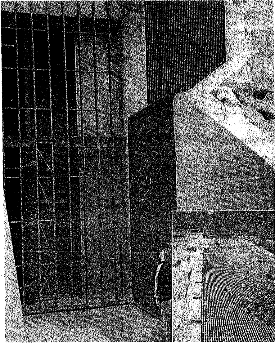
Figure 2.12 Pictured on the left are the steel trash racks on the fish exit of the Left Bank High Level Fishway at Hell's Gate. The widely spaced bars protect the fishway while the closely spaced bars protect the intake to the auxiliary water supply. The insert, lower right, shows the steel gratings on the fishway constructed at the site shown in Figure 2.10.
